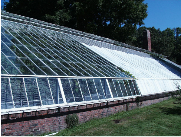
Figure 3.24. Lean-to style greenhouse at the Vale in Waltham. Note how almost the entire south façade is glazed, except for the short front knee wall. Lean-to style greenhouses like this used far more glass in their construction than the older conservatory style greenhouses.
