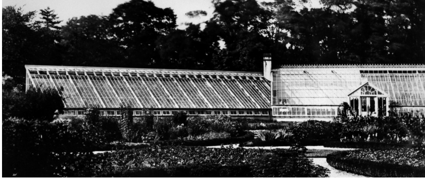
Figure 4.8. The greenhouses along the fruit wall at Gore Place, as they appeared in the early 20th century. They were built in a lean-to style, and may have reused architectural material from the 1806 greenhouse.
