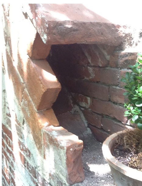
Figure 2.9. A brick flue that runs along the back wall of the 1804 greenhouse at the Vale. Part of this flue has been removed, making the interior visible.
