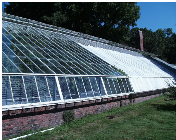
Figure 1.8. The lean-to style greenhouse at the Vale in Waltham. This example has a short front knee wall and a substantial back wall which support a south façade and roof made almost entirely of glass.
